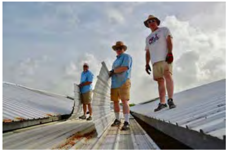
Bill Gerhart, Mike Albritton and Mark Moore repair a roof.
